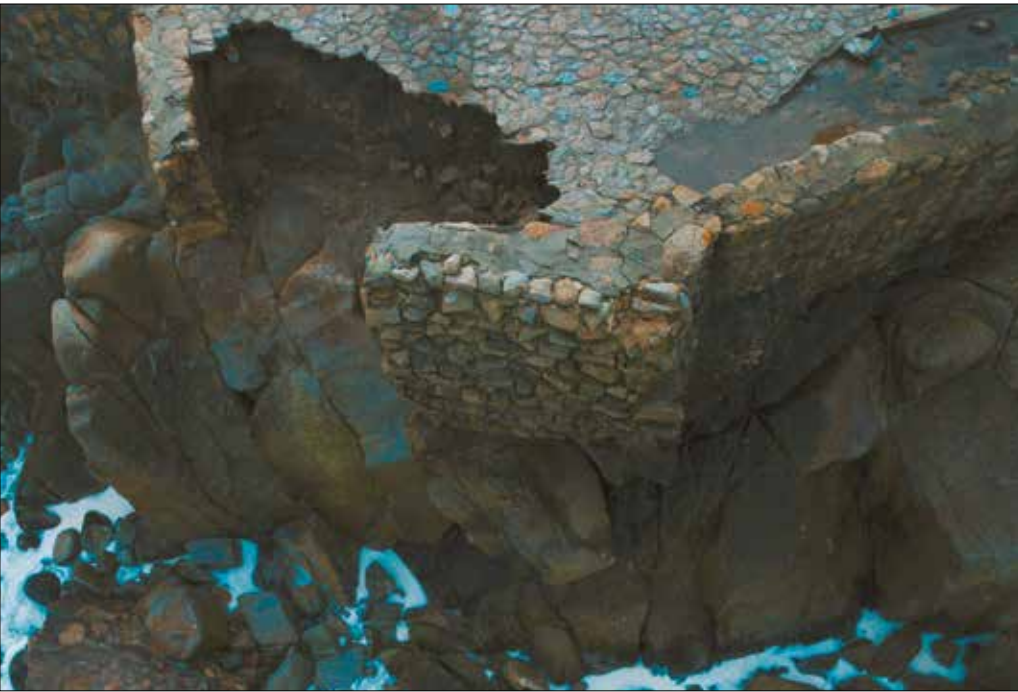
Above: Ryon Lane’s drone captured a photo of the broken sea wall on OceanView, clearly depicting the froth of the 20 to 30-foot waves pounding the shore. Below, the drone came in closer as the waves drew back and the damage can be seen.
